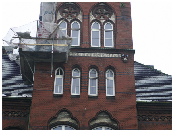
Fig. 10. Temporary steel-wooden platform and protecting nets.
