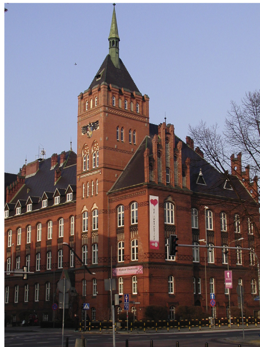
Fig. 13. General view of the renovated tower.
