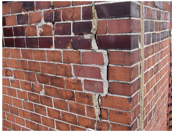
Fig. 5. Dislocated part of the newly built-in bricks (on the stiff cement mortar).
