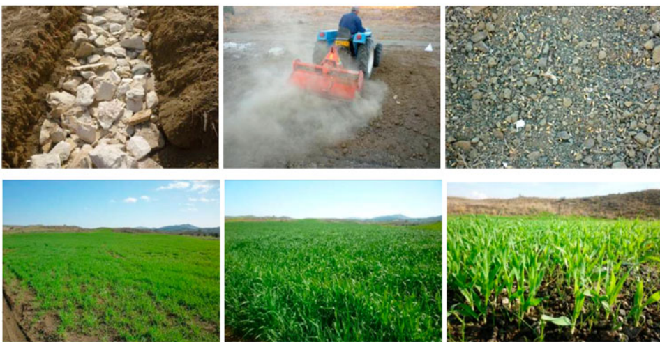
Figure 3. The test field in Alampra village during its construction, cultivation and barley growth.
